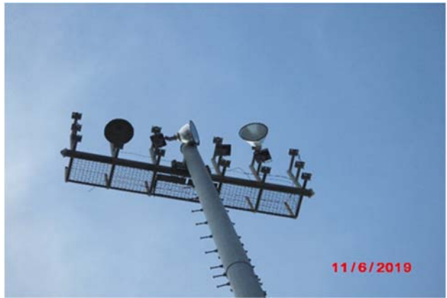
The three (3) existing 1500-watt spotlights on metal pole at the southeast corner of the track and field.
