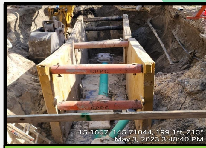
INSTALLATION OF 12" SEWER PIPE AND LATERAL STUB OUT.
