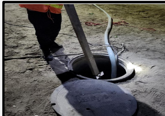
LAMP TEST FOR THE NEW SEWER MANHOLE 1 AND 2
