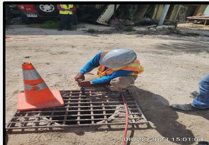
PRESSURE TEST FOR THE NEW SEWER MANHOLE 1 AND 2
