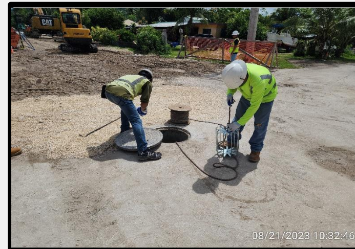
MANDREL TEST FOR THE NEW SEWER MANHOLE 1 AND 2
