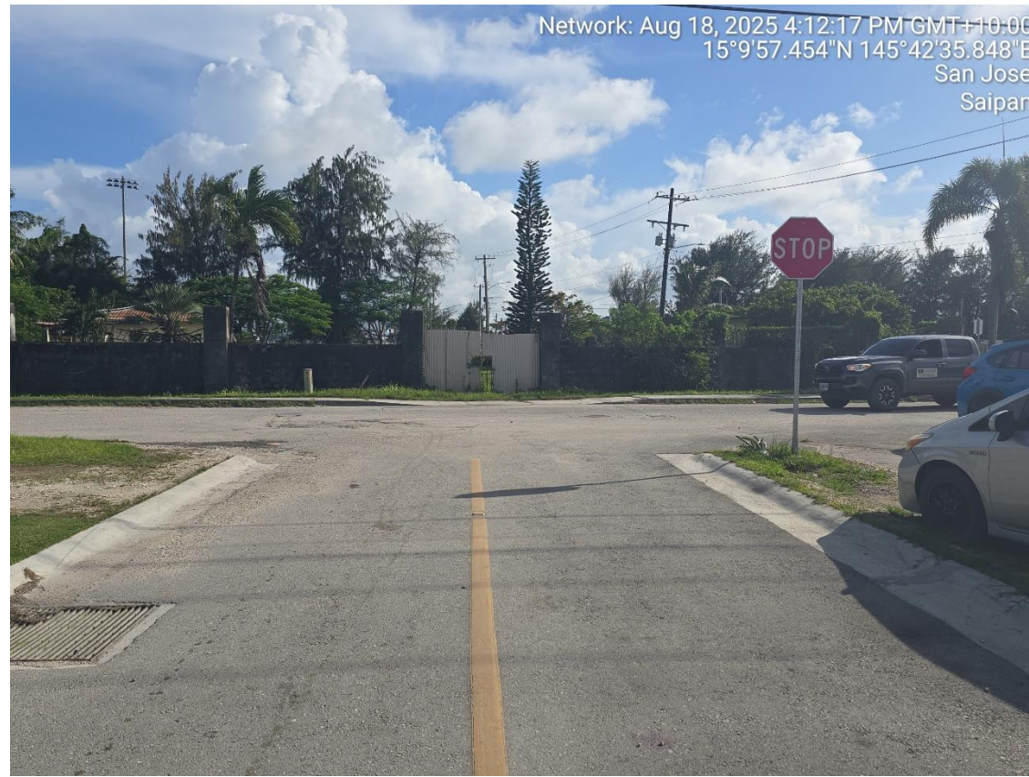
START OF THE PROJECT AT APENGAGH AVENUE
