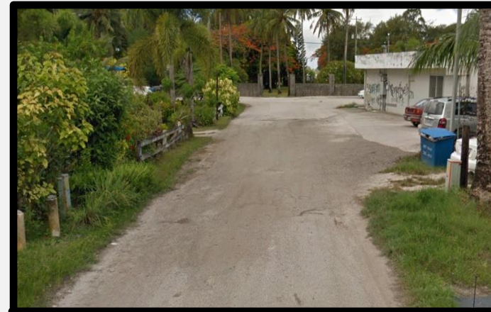
OLD ASPHALT ROADWAY (LOCATION OF THE NEW SEWER MANHOLE 2) IN FRONT OF RNV APARTMENT ALONG APENGAGH STREET (GOING SOUTH).
