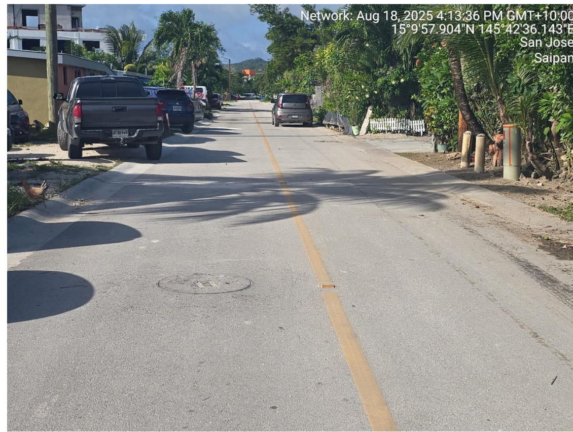
NEW SEWER MANHOLE 2 ALONG APENGAGH AVENUE
