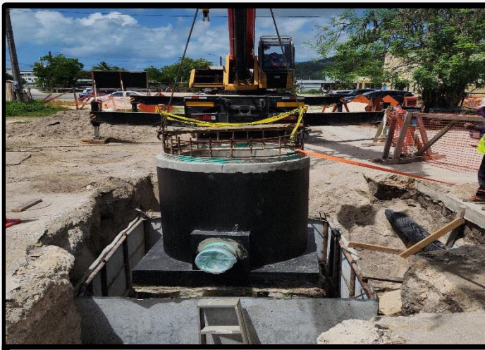
LIFTING AND INSTALLING OF NEW CONCRETE SEWER MANHOLE 1
