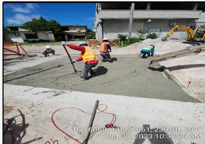
CONCRETE ACTIVITIES FOR THE FLOWABLE FILL
