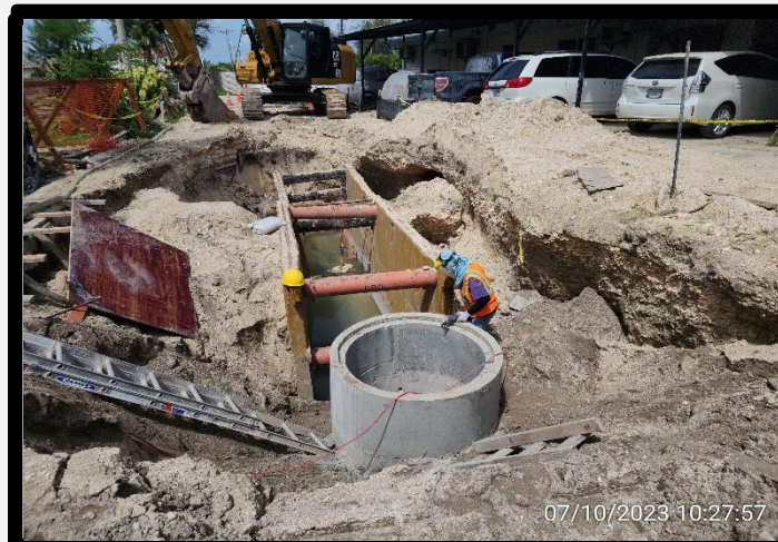
LIFTING AND INSTALLING OF SEWER MANHOLE 2.
