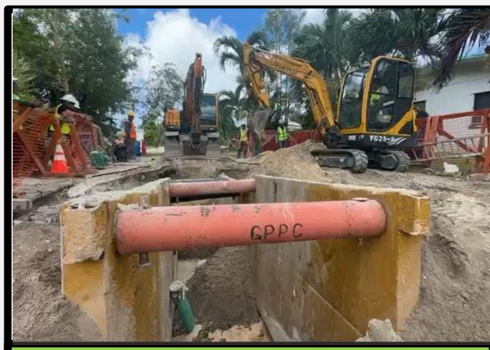
EXCAVATION AND INSTALLATION OF TRENCH SHIELD.
