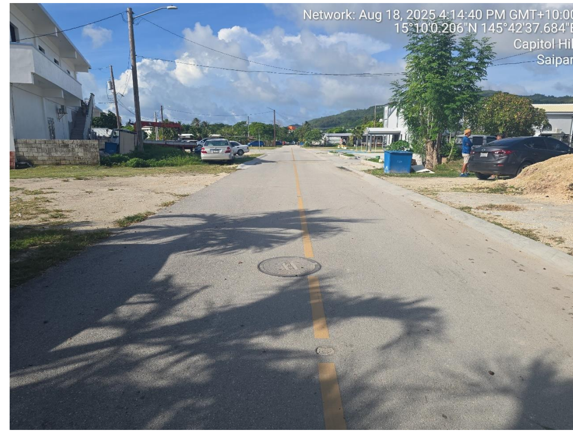
NEW SEWER MANHOLE 1 ALONG APENGAGH AVENUE
