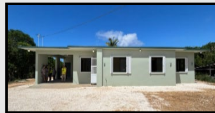
4 Bedroom New Construction
