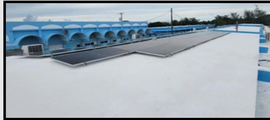
Tinian Elementary School rehab Phase II
