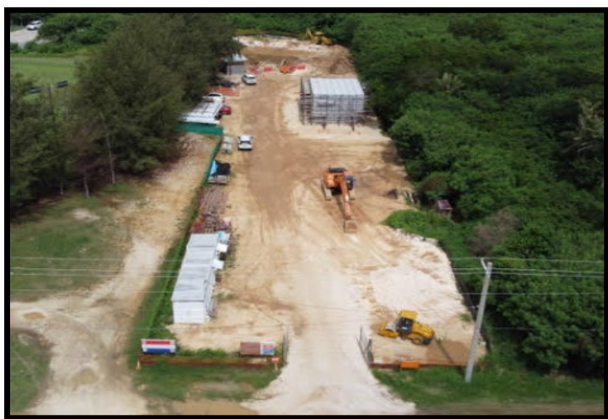
Dandan Water Tank Project Site
